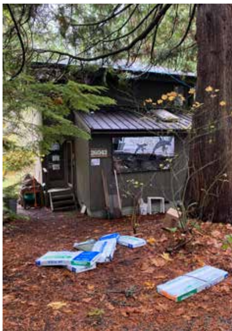
The Stillwaters Tree House about to receive a new roof.
